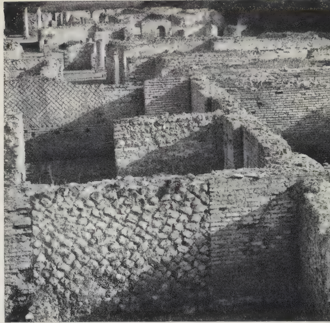
Examples of opus incertum , opus reticulatum , and brick facing
